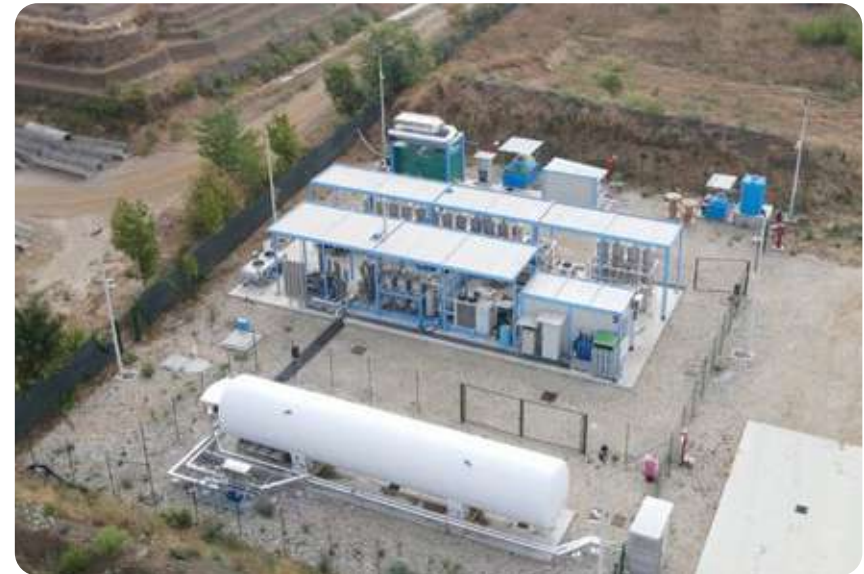
Novi Ligure - Landfill managed by SRT S.p.A Biogas upgrading + biomethane liquefaction & storage
